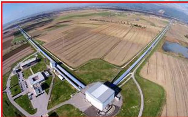
**Air pressure on the vacuum tubes:** 155-million kg (341-million pounds) of air press down on each 4 km length of vacuum tube. Remarkably, the steel tubes that hold all that air at bay are only 3 mm (0.12 inches) thick.
