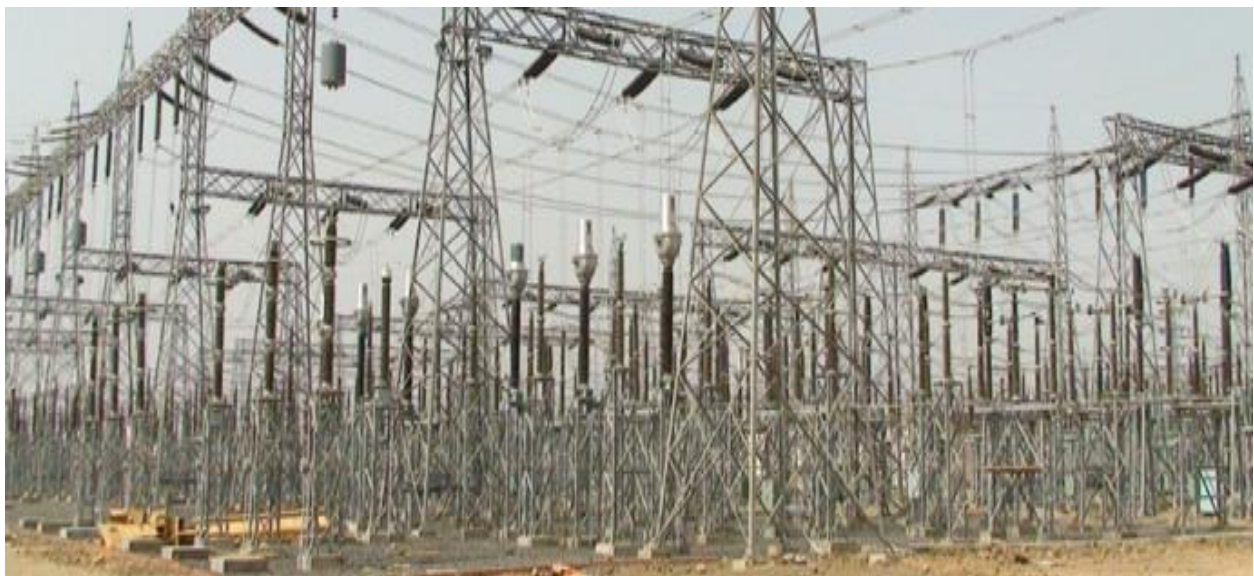
View of 220kv Receiving Substation, GETCO, Nasari
